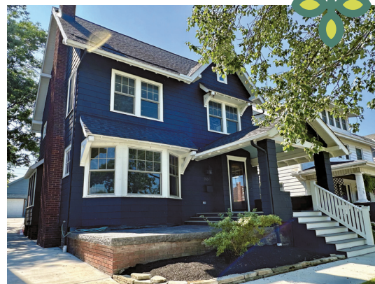
1462 Belle Ave. This classic Arts and Crafts home with its welcoming porch was saved and rehabilitated after a house fire.
